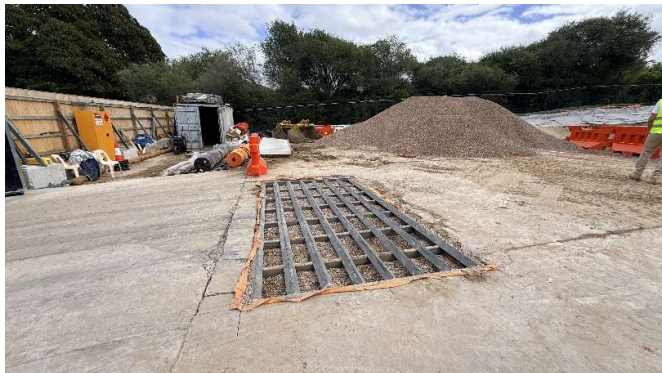
Photo 11: Northern boundary – Concrete pad and rumble grid installed at the site access/egress point. The area was observed to be clean at the time of inspection.
