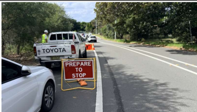
Photo 12: Public road – Traffic control signage installed along surrounding public roads approaching the site access/egress point.
